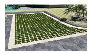
Grass blocks are an interlocking cavity grid system that offers natural looking hard standing for vehicles and can be an excellent alternative to plain concrete surfaces for parking lots, driveways, and access roads for vehicles. Grass blocks can also be used for erosion control.
