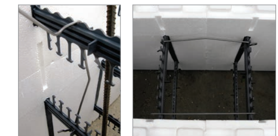
Vertical Clips in Place Horizontal Clips in Place Note: You can skew the HV Clip a notch or two for an even tighter fit, if needed.
