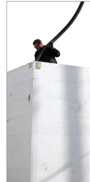
The Fox Blocks extended 90° corner block showing it's stand alone strength during concrete placement.
