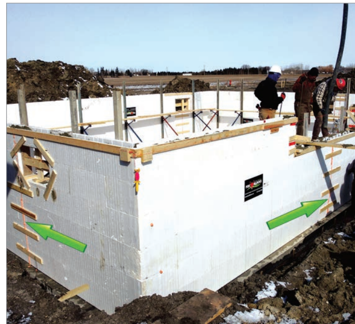
Here is a job, post concrete, that has been constructed exactly to the building dimension by properly stacking seams.
